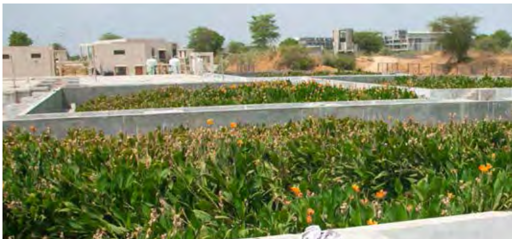
Figure 24. The Canna indica plant, used in the Planted Gravel Filter (PGF), a critical step in the sewage treatment process
