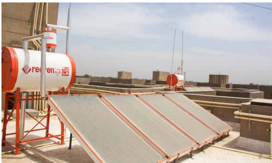
Figure 30. Solar water heater tank with solar panels in Housing
