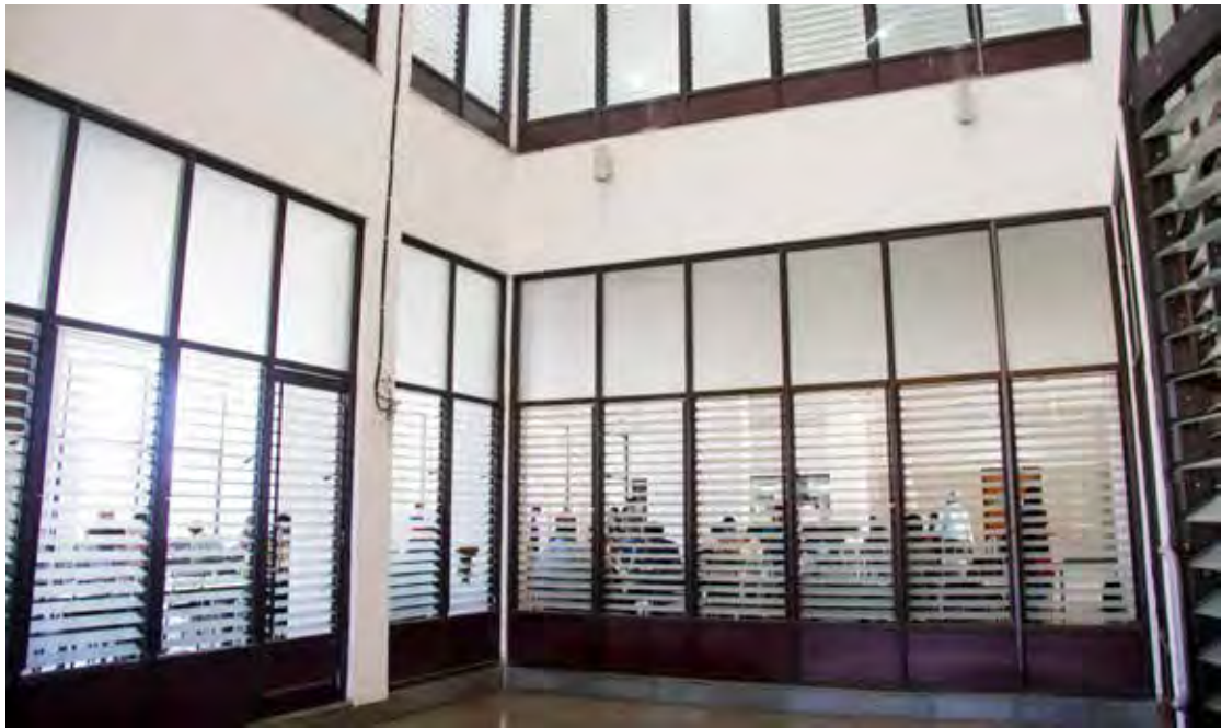
Figure 31. Shaft for the Passive Downdraft Evaporative Cooling in the student hostel mess
