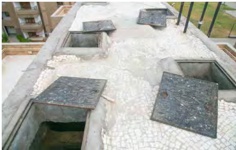
Figure 10. Rooftop storage tank with separate chambers for fresh and recycled water
