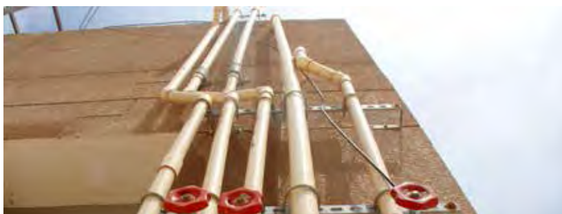
Figure 11: Different pipes for firefighting, clean water, recycled water, rainwater from housing roof
