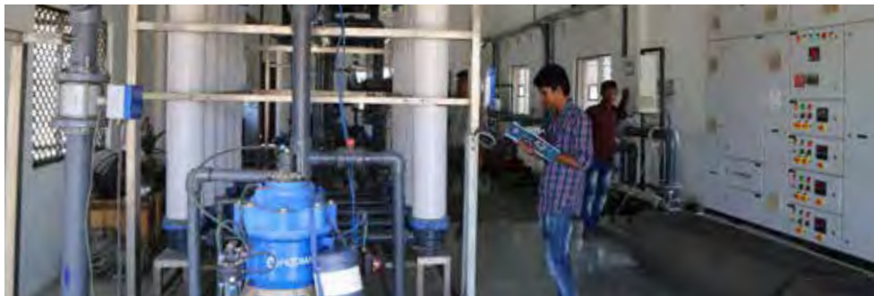
Figure 1. Ultra filtration Unit
