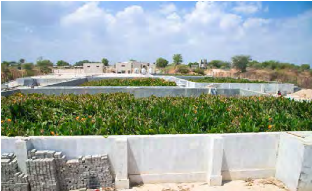
Figure 6. Root Zone treatment system where Canna indica plant roots help to treat the effluent
