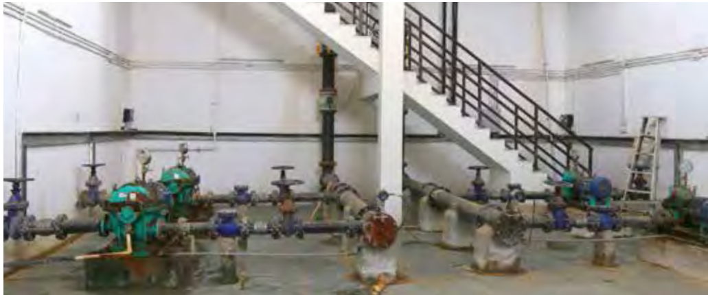
Figure 9: Typical pumping arrangement at a WSC: pumping and distribution system for fresh and recycled water
