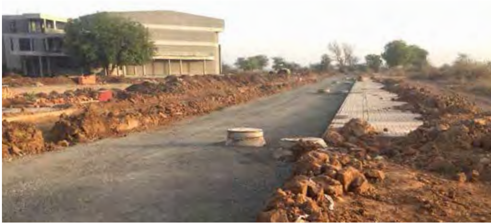
Figure 14. Masonry manholes under construction
