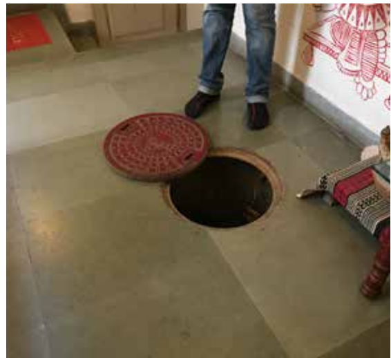
d) Water accessed by lifting cover of cistern
